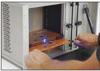
Installing an output expansion switch blade
